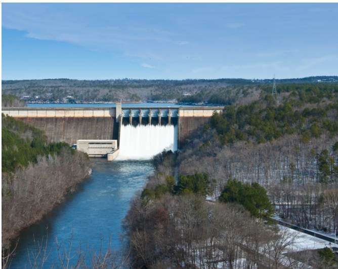
Dam at Greers Ferry
