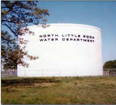
A water tank of the City of North Little Rock Water Department.
