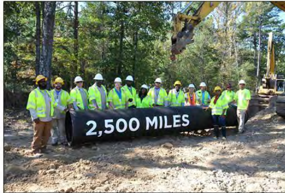
CAW installed its 2,500 th mile of pipe in 2017.
