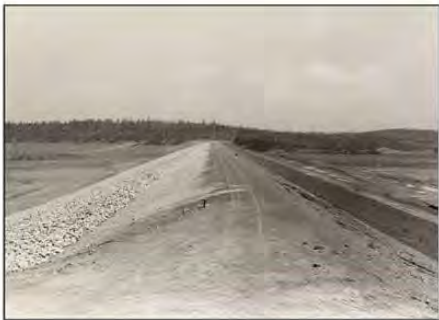
1957 – Lake Maumelle construction.
